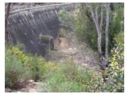
concrete wall. With more heavy rains forecast Barwon Water closes scour valve to halt movement of sediment from reservoir – and reservoir refills. They temporarily retro-fit new valve to old valve which then can remain open with water levels in the reservoir being managed via the new valve.
