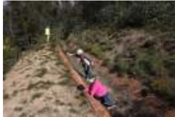
Cook children doing a serious inspection of the Aqueduct condition
