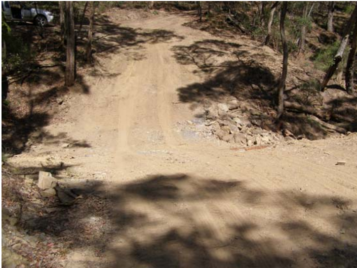
Re establishment of the Red Ironbark Tk Crossing
